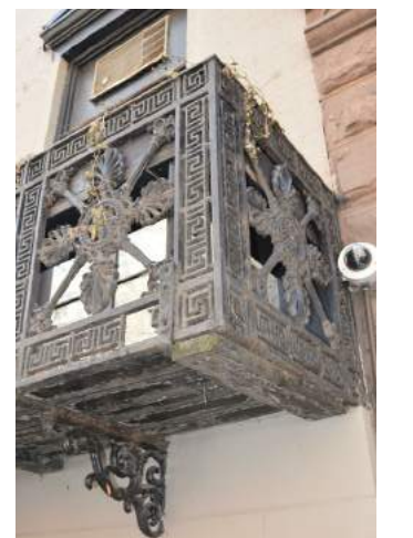
PROPOSE TO REPAIR RUST AND REPAINT THE BALCONY
