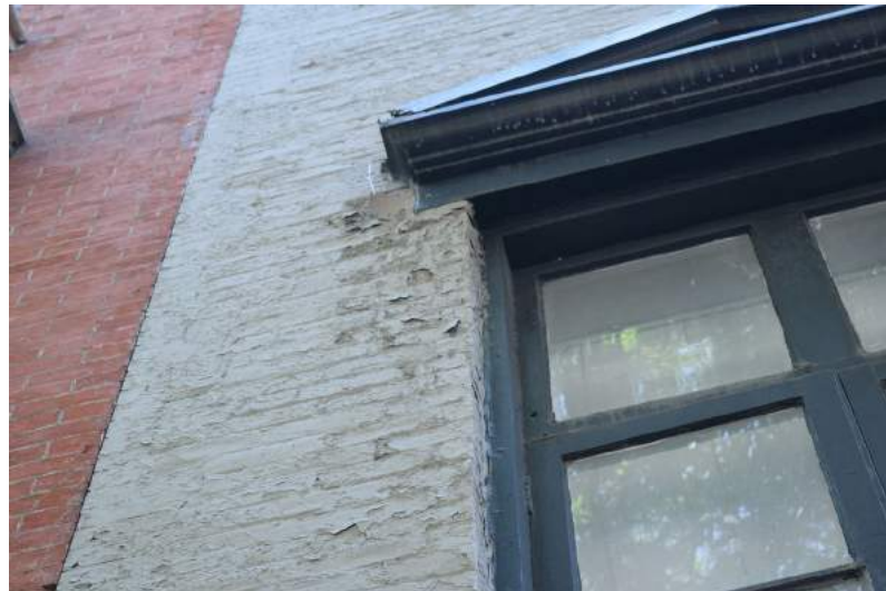
EXISTING BRICK CONDITION PROPOSING TO REMOVE PAINT AND REPOINT
