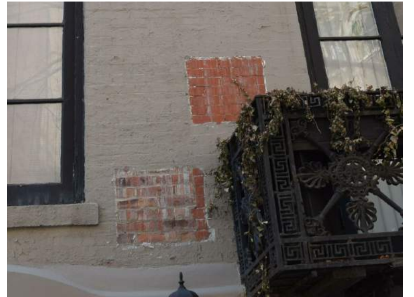
EXISTING BRICK CONDITION PROPOSING TO REMOVE PAINT AND REPOINT
