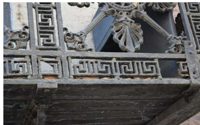
EXISTING CONDITION OF BALCONY WHICH NEEDS TO BE REPAINTED AND REPLACE THE MISSING DECORATIVE ORNAMENTS
