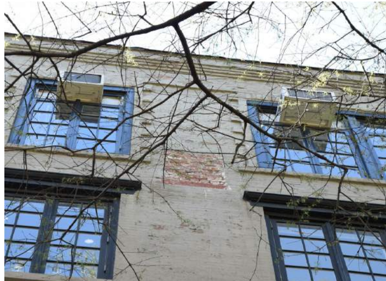
EXISTING BRICK CONDITION PROPOSING TO REMOVE PAINT AND REPOINT
