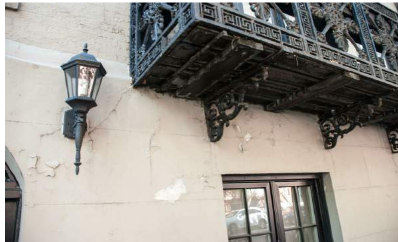
EXISTING CONDITION OF BUILDING BASE. PROPOSE TO COVER IT WITH BROWNSTONE
